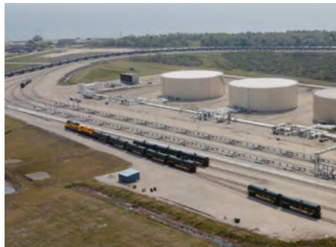
USDG's Port Arthur Terminal, in Port Arthur, Texas (the DBR network destination terminal).
